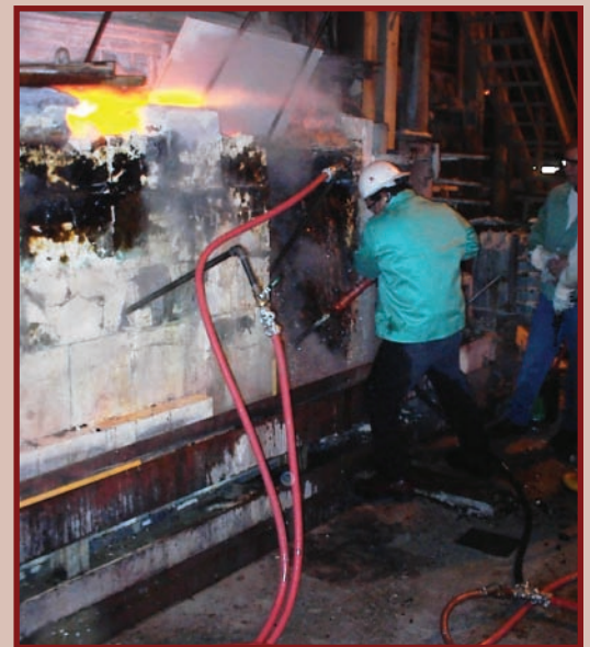
Hot Doghouse Replacement
